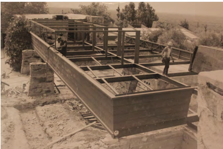
Figure 6-17 - Reconstruction of the Guest Deck in 1970 (The Frank Lloyd Wright Foundation Archives, The Museum of Modern Art | Avery Architectural & Fine Arts Library, Columbia University, New York).
