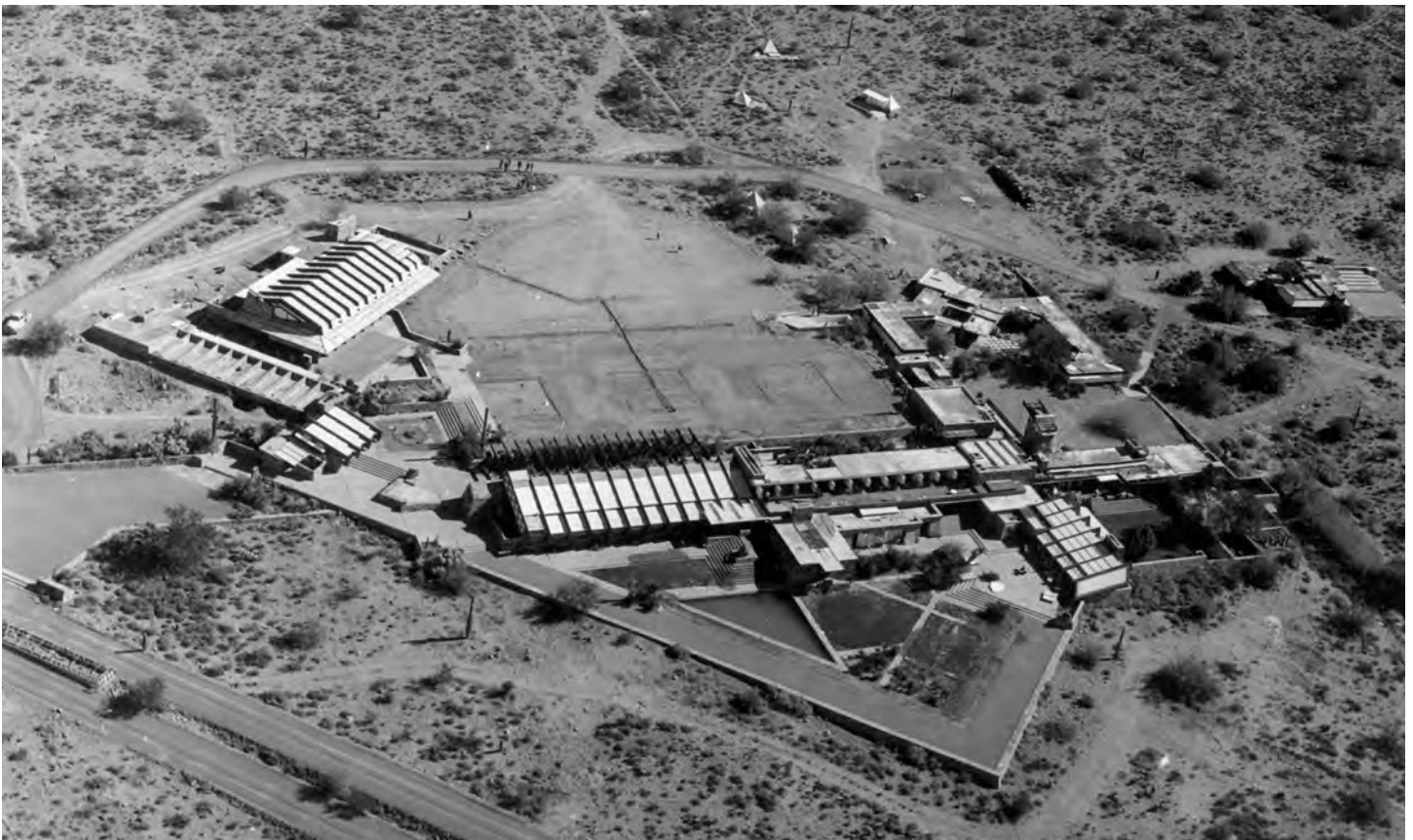
Figure 10-1 - Aerial view of Taliesin West, 1959 (Pedro Guerrero).
