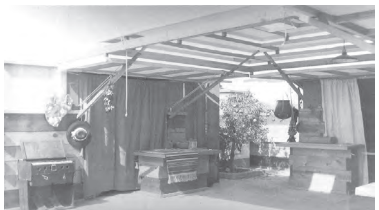
Figure 6-10 - Interior of Sun Trap, ca. 1939 (The Frank Lloyd Wright Foundation Archives, The Museum of Modern Art | Avery Architectural & Fine Arts Library, Columbia University, New York).
