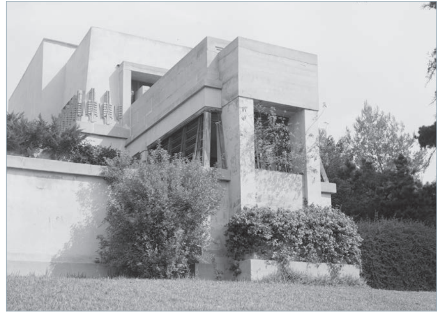
Hollyhock House, view of south elevation, September 1965. Photograph by Marvin Rand, Library of Congress, Prints and Photographs Division, Historic American Buildings Survey, Reproduction number HABS CAL,19-LOSAN,28-5.
