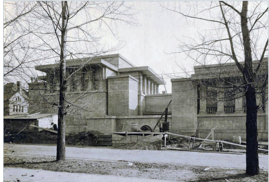
Unity Temple, view of west elevation during construction, 1909.
