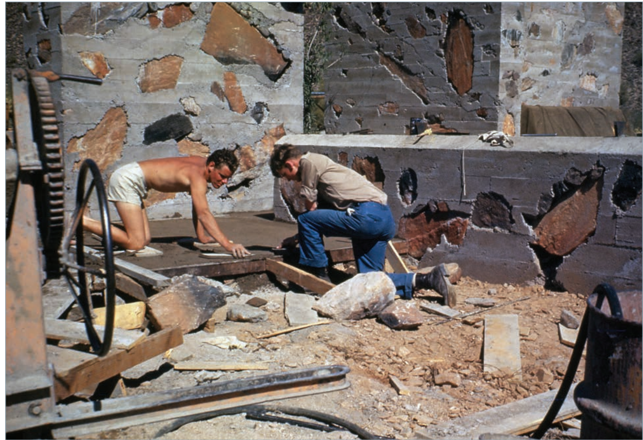
Taliesin West, apprentices constructing cabaret theater, 1949.
