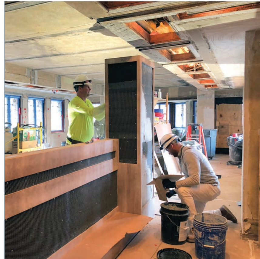
Robie House, recreation of missing inglenook bench, 2018
