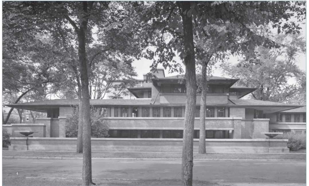
Frederick C. Robie House, view looking south, August 1963. Photograph by Cervin Robinson, Library of Congress, Prints and Photographs Division, Historic American Buildings Survey, Reproduction number HABS ILL,16-CHIG,33-4
