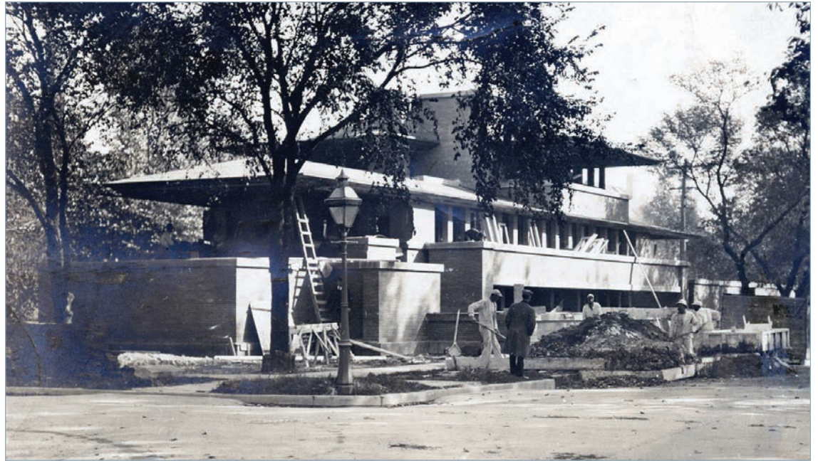
Frederick C. Robie House, view of south elevation during construction, 1909. Photograph courtesy of the Frank Lloyd Wright Trust.
