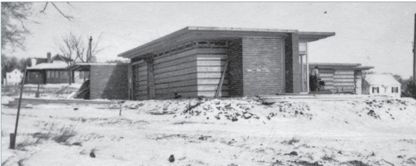
Herbert and Katherine Jacobs House, view of street elevation looking northeast, circa 1937. Photograph by John H. Howe, courtesy of the Wisconsin Historical Society, WHS-25609.
