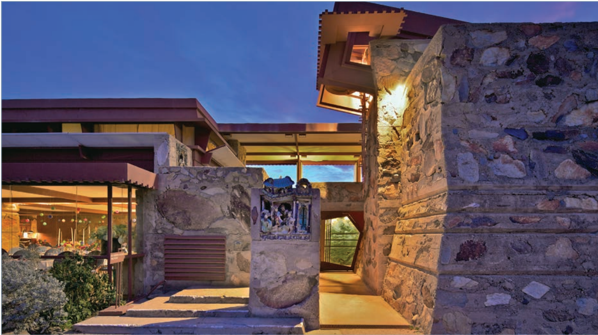
Taliesin West, view to the south showing entrance door leading to dining room (left) with guest deck apartments (above), and desert masonry structure of kitchen (right).
