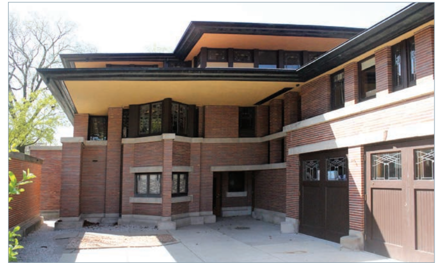
Frederick C. Robie House, view of south elevation showing main level's south prow and its cantilevered roof eaves, third floor bedroom level, and courtyard with staff quarters over former garage (now museum gift store). Photograph courtesy of Harboe Architects.
