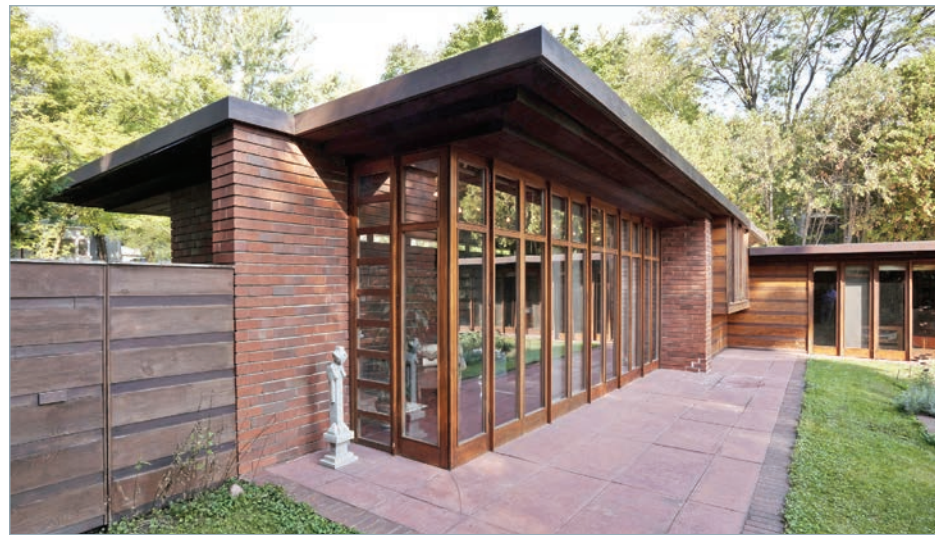
Herbert and Katherine Jacobs House view to the northwest of living room corner door and “Cherokee” red pigmented concrete slab on interior floor and exterior terrace.
