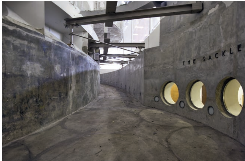
The Guggenheim Museum's Sackler Center for Arts Education, located beneath the spiral rotunda, offered close-up views of the preservation work, May 2005. The museum's circular grid is visible on the floor and mimicked in elements such as the windows into the Sackler Center, the lighting fixtures between them. Photograph by David Heald, courtesy of the Solomon R. Guggenheim Foundation.
