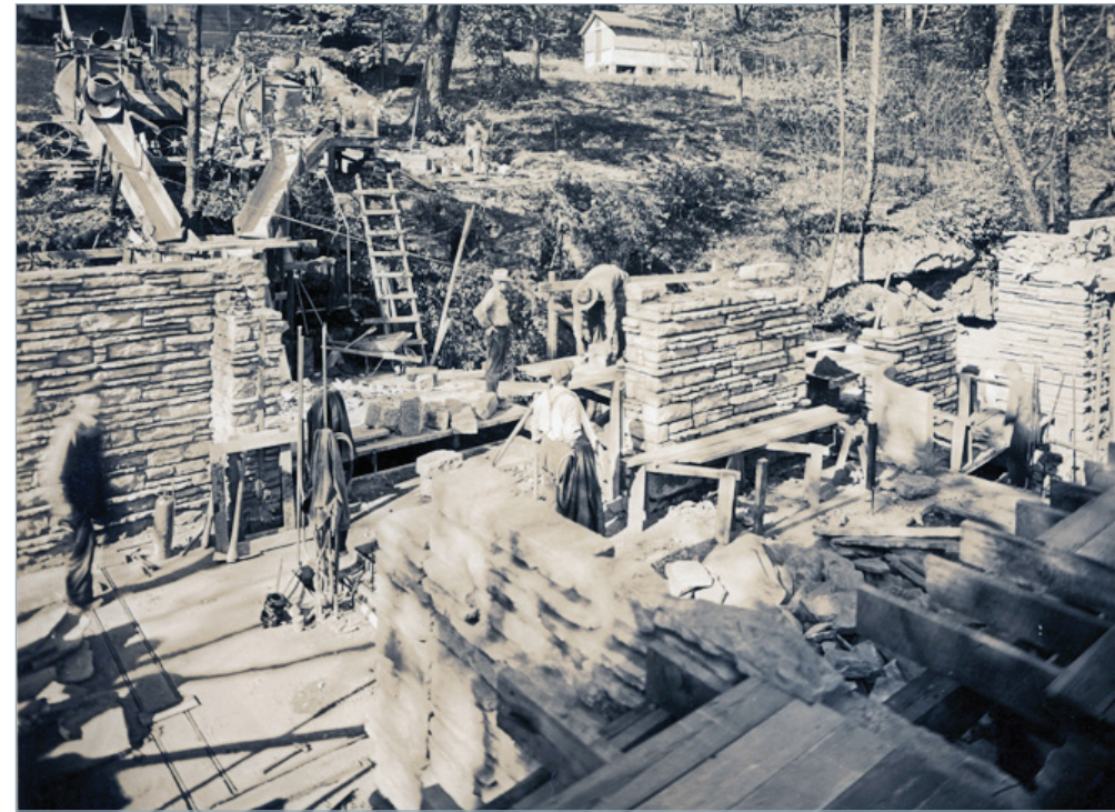
Fallingwater, view showing construction, facing north, circa 1936.
