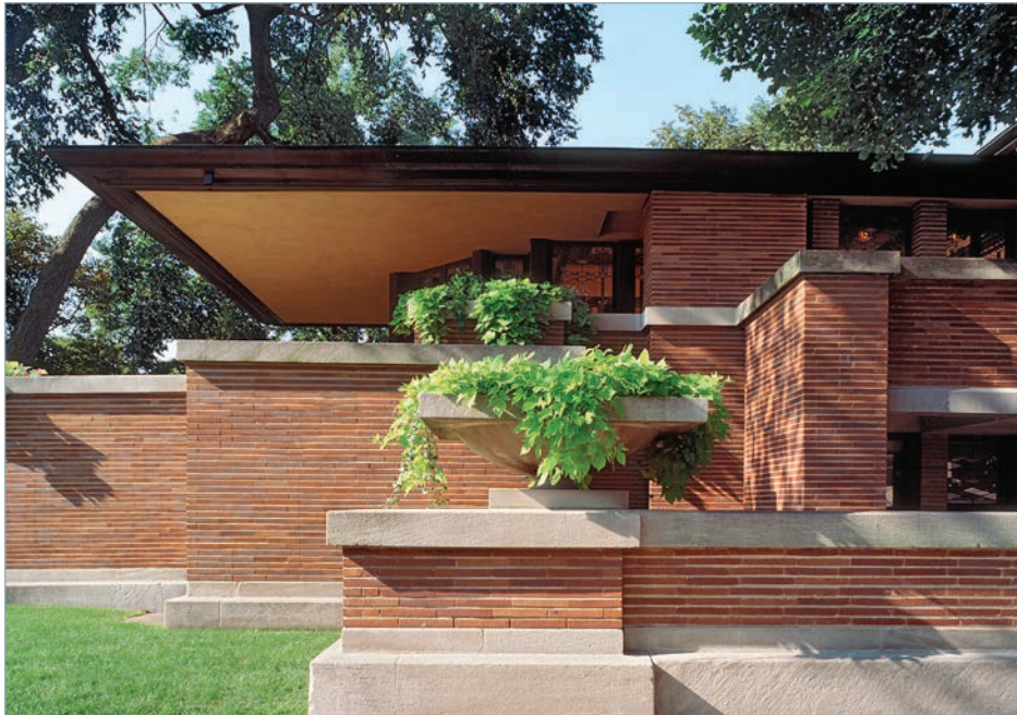
Frederick C. Robie House, view showing cantilevered roof eaves over porch at northwest corner and raked Roman brick piers capped with limestone. Photograph courtesy of the Frank Lloyd Wright Trust.
