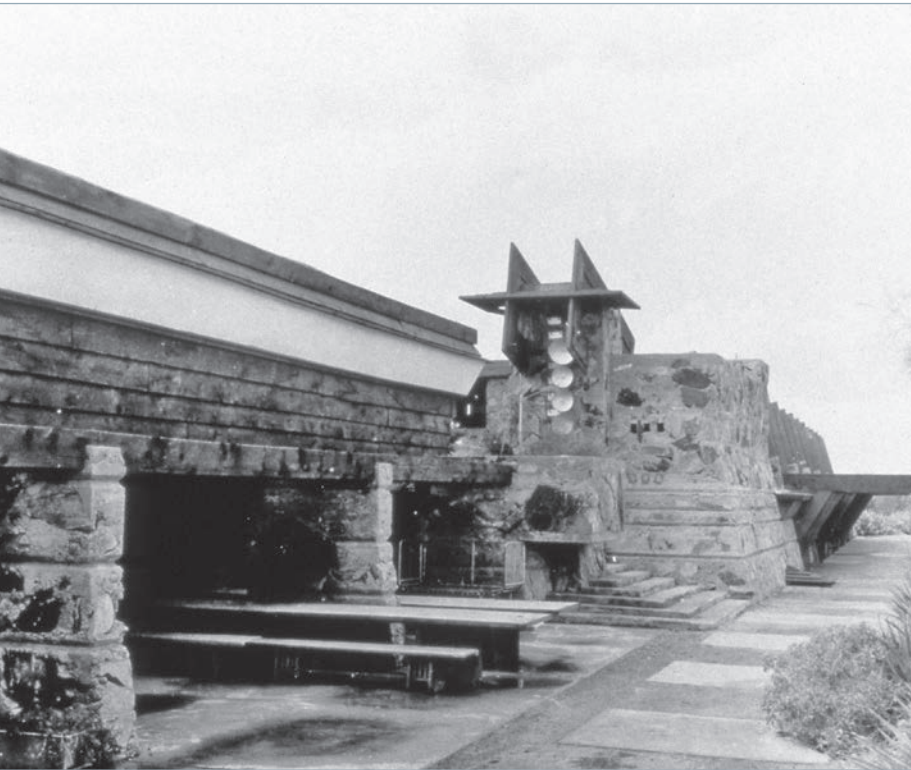
Taliesin West, view of dining loggia with drafting studio beyond, 1939. The Frank Lloyd Wright Foundation Archives (The Museum of Modern Art | Avery Architectural and Fine Arts Library, Columbia University, New York), 3803.3731.
