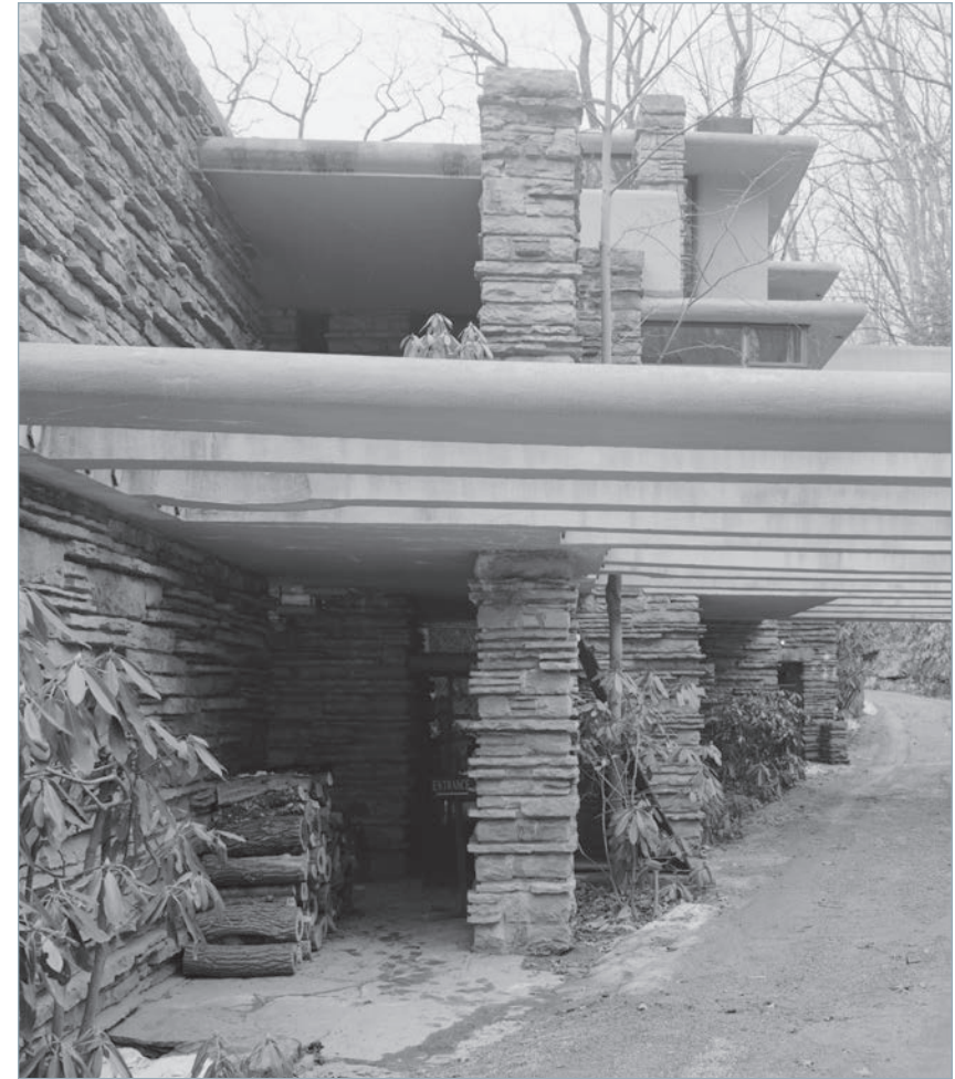
Fallingwater, view of trellis beams over main entrance to house, 1985. Photograph by Jack E. Boucher, Library of Congress, Prints and Photographs Division, Historic American Buildings Survey, Reproduction number HABS PA,26-OHPY,V,1-22.
