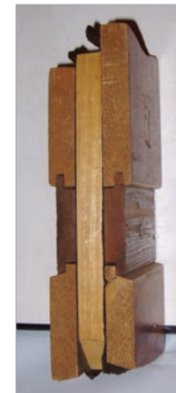
Herbert and Katherine Jacobs House, sample of "sandwich wall" construction.
