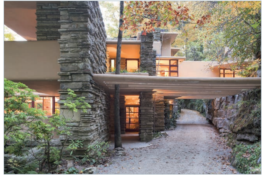
Fallingwater, view of entry (center) with trellis beams extending across drive. Photograph by Christopher Little, courtesy of the Western Pennsylvania Conservancy.
