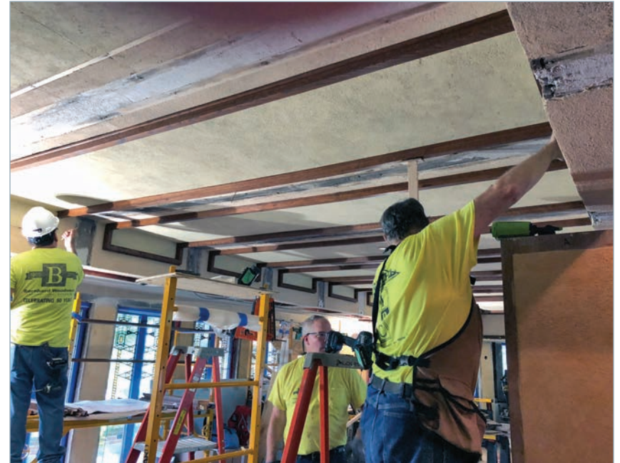
Robie House, restoration of guest bedroom plaster, 2018
